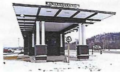
Passenger canopy was rebuilt as part of the restoration
