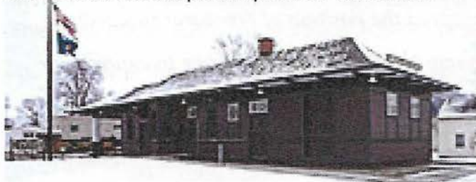
The restored and adapted depot after restoration
